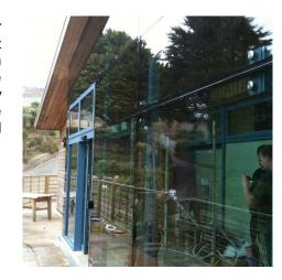
polyester powder coated perimeter channel frame fitted back to the existing structure and to a new steelwork frame fixed to the slab and glulam roof beams.
